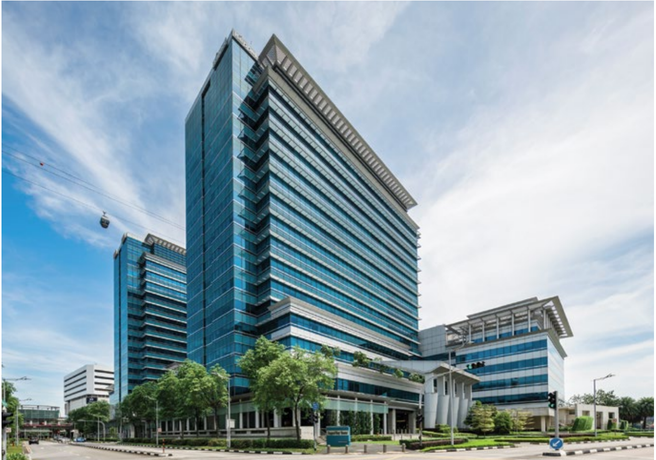
Energy-efficient technologies were piloted at Keppel Bay Tower under BCA's Green Buildings Innovation Cluster (GBIC) programme. Image: Keppel.
