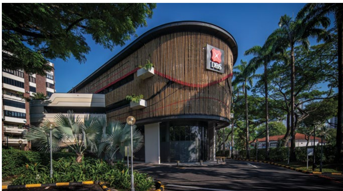
DBS Newton Green has been certified as a Green Mark Platinum Zero Energy building. Image: DBS Bank Ltd.
